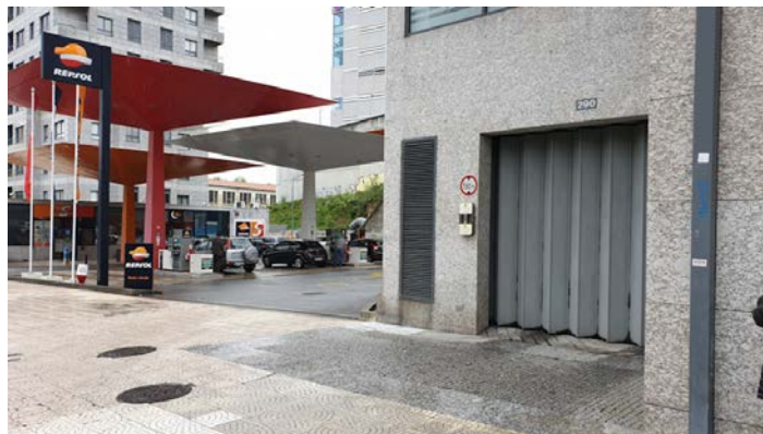
Figure: parking gate.
